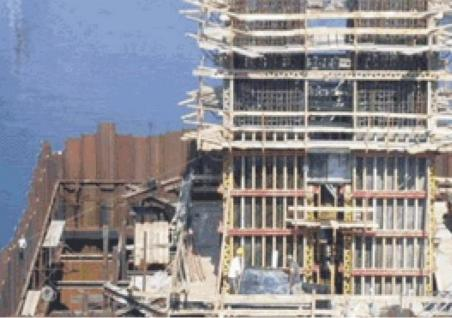
Prestressed concrete structure of variable edge built by successive cantilever procedure with the use of 5 tn blondín as an auxiliary element
